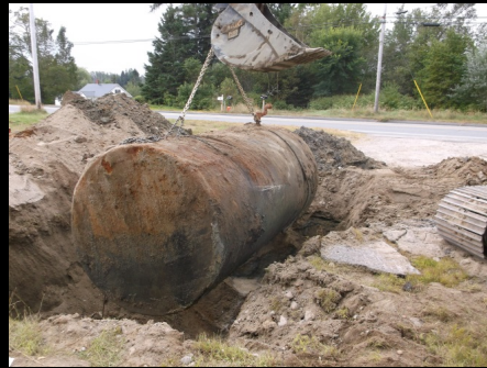
Test pits & gasoline tank removal, Harrington
