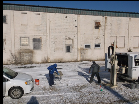
GeoProbe soil borings, Eastport
