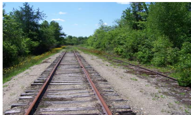
Figure 5-19 Charlotte Siding to the Right
