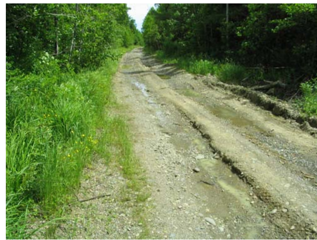
Figure 5-32 Rutting due to Logging Operations
