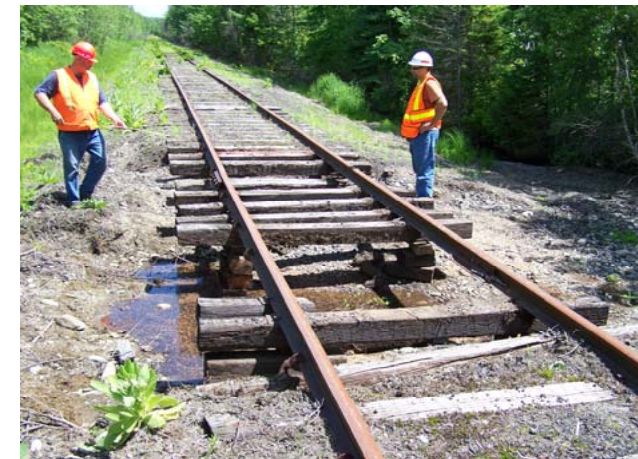
Figures 5-23 and 5-24 Two of the Washouts between MP 256.6 and 256.9
