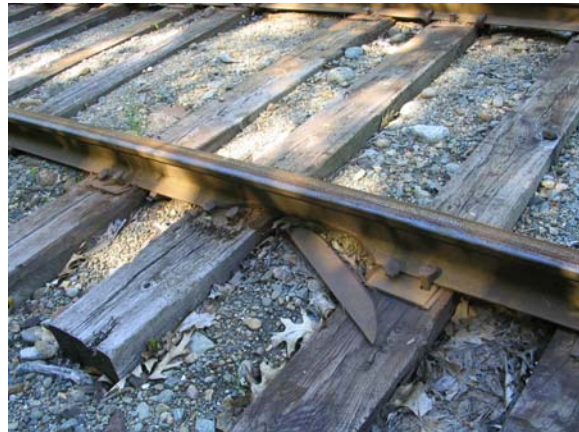
Figure 5-12 Broken rail base in 75# Rail
