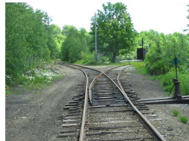
Figure 5-10 No. 5 Frog Turnout at Milltown Jct. Looking South. Salmon Falls Br. 269.02 to NBSR is to the Right.
