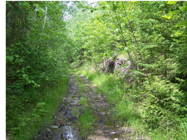
Figure 5-33 Wet Area in Rock Cut
