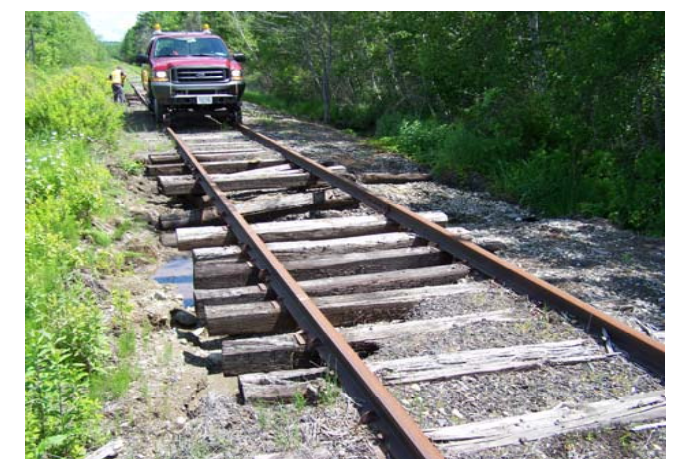
Figures 5-23 and 5-24 Two of the Washouts between MP 256.6 and 256.9
