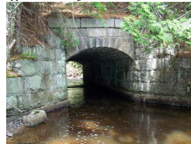
Figure 5-35 Stone Box Culvert
