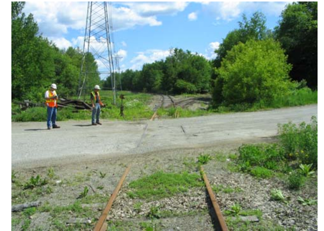
Figure 5-5 Private Crossing near Woodland Jct. Note turnout that is north end of Wye
