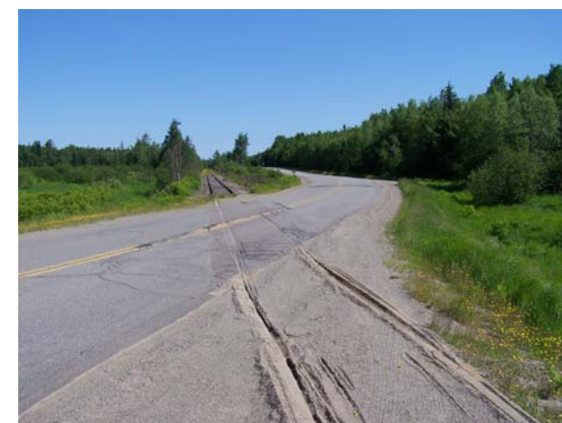
Figure 5-28 Charlotte Road Crossing
