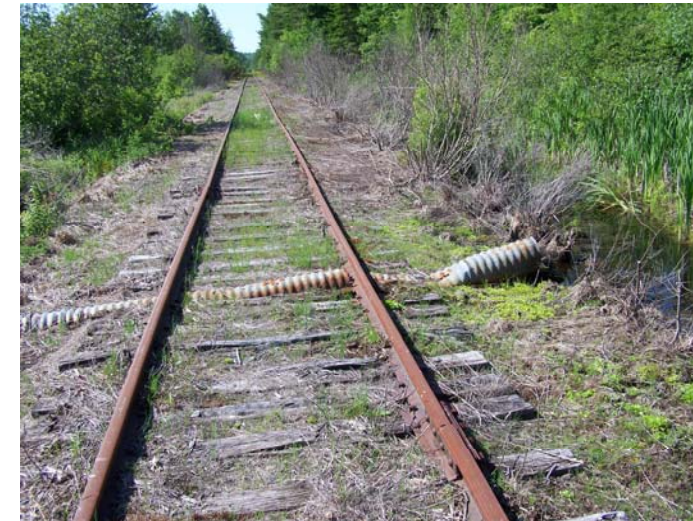
Figure 5-25 Crushed CMP Pipe at MP 261.67
