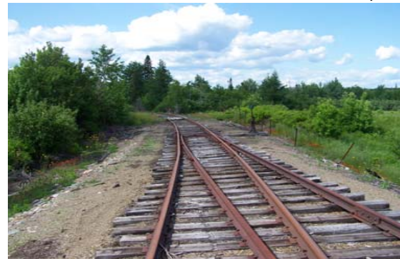
Figure 5-20 East Main Track Switch Ayers Jct.
