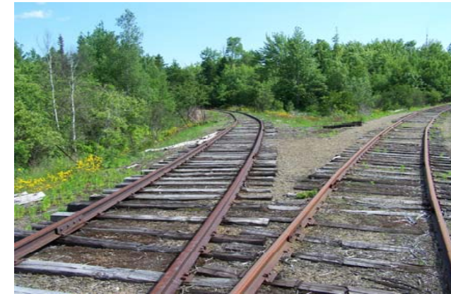
Figure 5-21 Ayers Jct. East Main Switch Behind Camera
