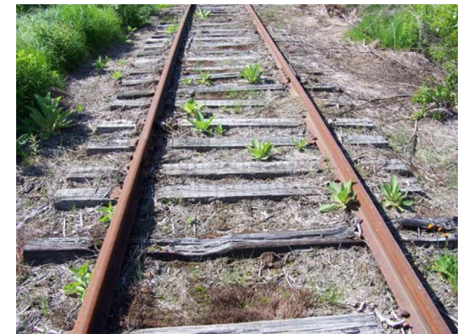
Figure 5-15 Close up of Tie Condition
