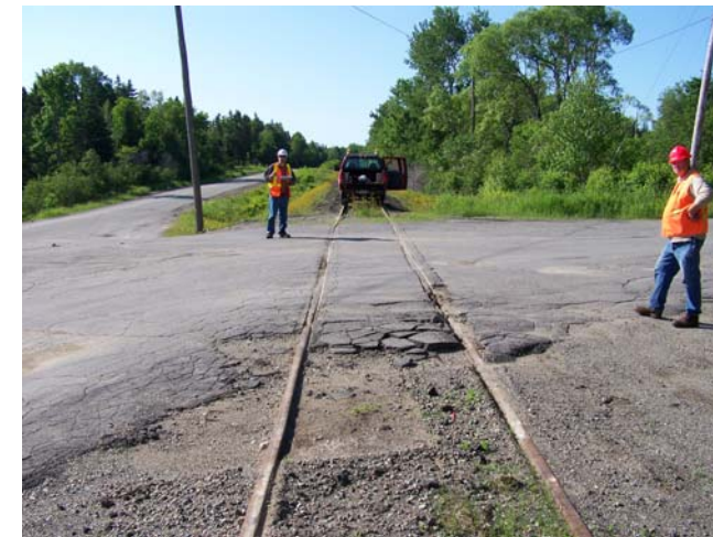
Figure 5-26 Lane's Construction Crossing
