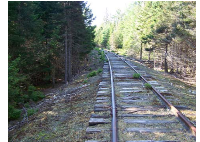
Figure 5-17 Track on Fill Section Wetland
