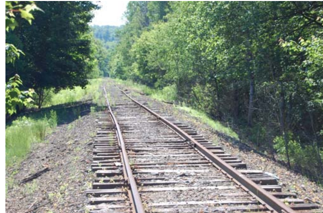
Figure 5-13 Typical Track Conditions in Canadian Segment
