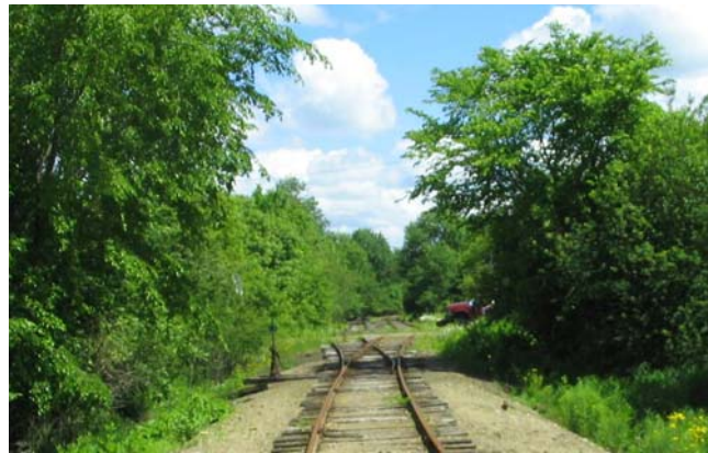
Figure 5-6 Turnout, Siding and Reverse Curve at Baring.
