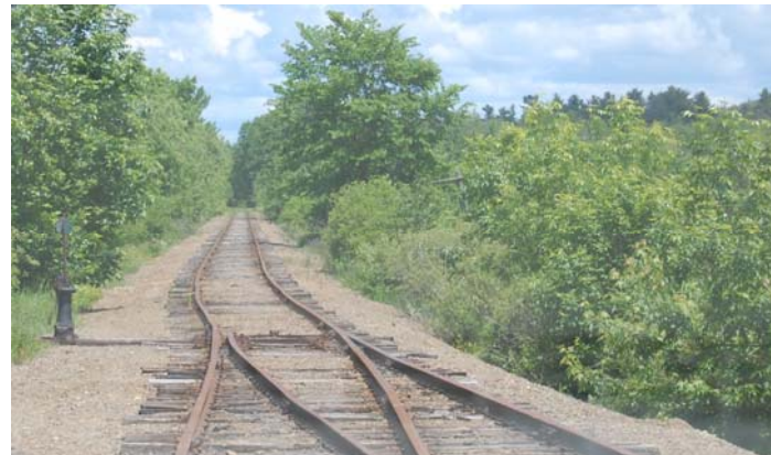
Figure 5-7 St. Croix Junction, Looking Towards Calais. Note Reverse curve due to Placement of Turnout in Curve to Track to the Right
