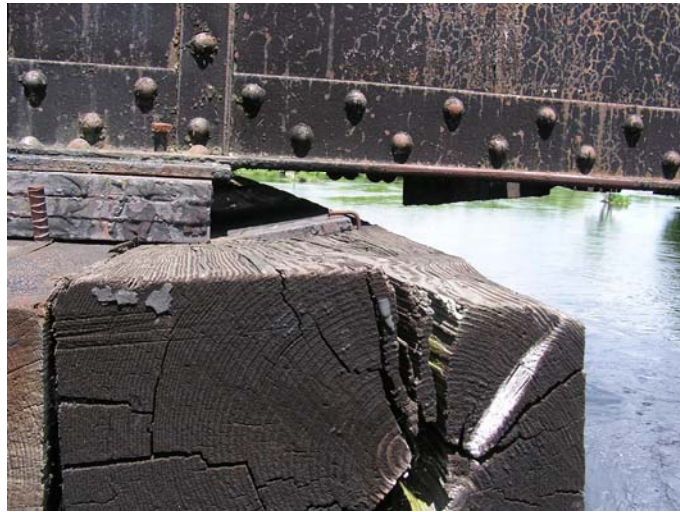
Figure 6-11 Baring International Bridge. Note rotated shims and new steel added to girder.
