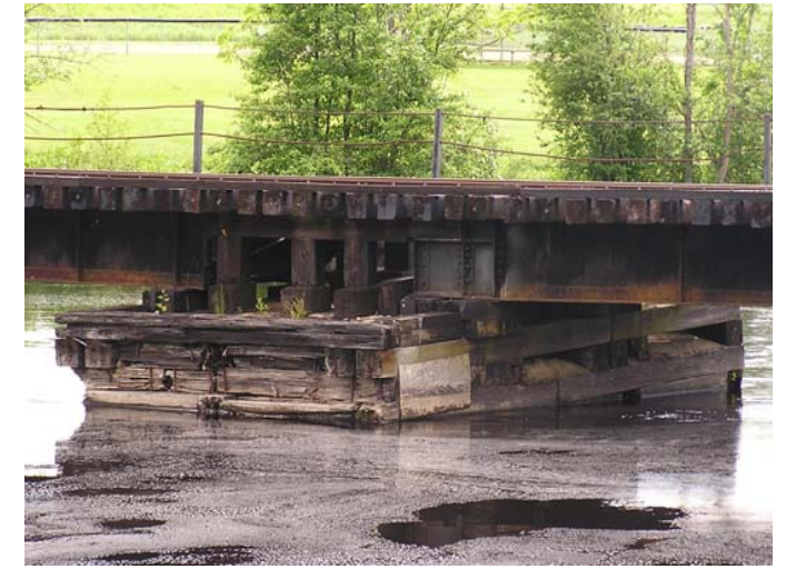
Figure 6-14 Salmon Falls International Bridge. Note uneven timber cribbing which supports the steel girders.
