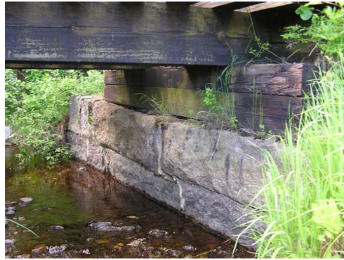
Figure 6-18 Bridge Over Moosehorn Brook. Note loose shims and vegetation growth at abutment seat.
