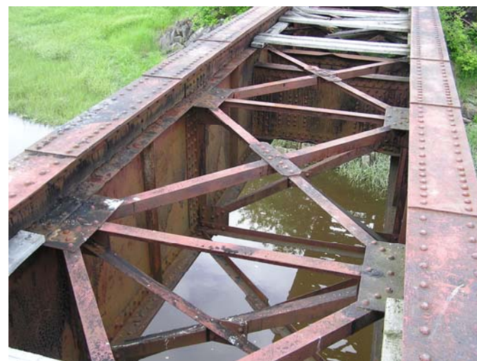
Figure 6-36 Bridge Over Little River, top of deck.
