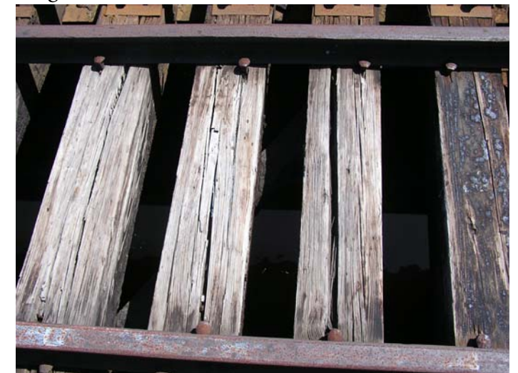
Figure 6-04 Sprague Falls International Bridge. Note typical deterioration to timber ties.
