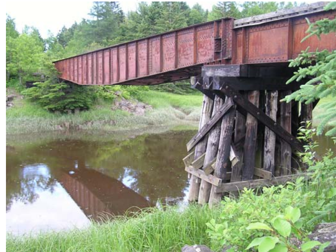
Figure 6-34 Bridge Over Little River, main span and timber pier support.
