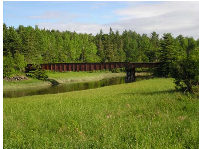
Figure 6-33 Bridge Over Little River looking south.
