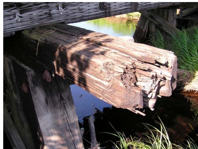
Figure 6-27 Bridge Over Ohio Brook. Note severe deterioration at end of pile cap which continues throughout the length of the member.
