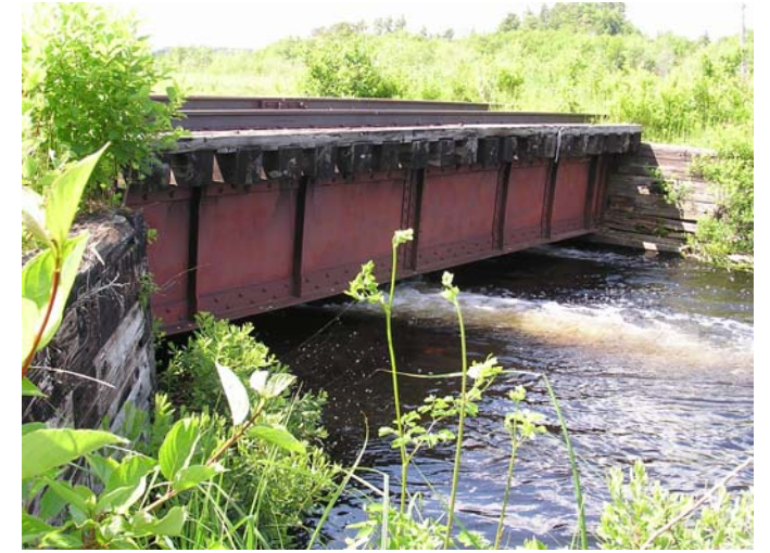
Figure 6-22 Bridge Over Round Pond Stream. Note high water flow due to beaver dam on opposite side.
