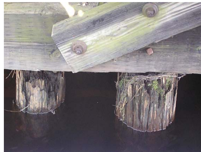
Figure 6-28 Bridge Over Ohio Brook. Note the deterioration at the top of the piles which result in reduced/non-bearing conditions.
