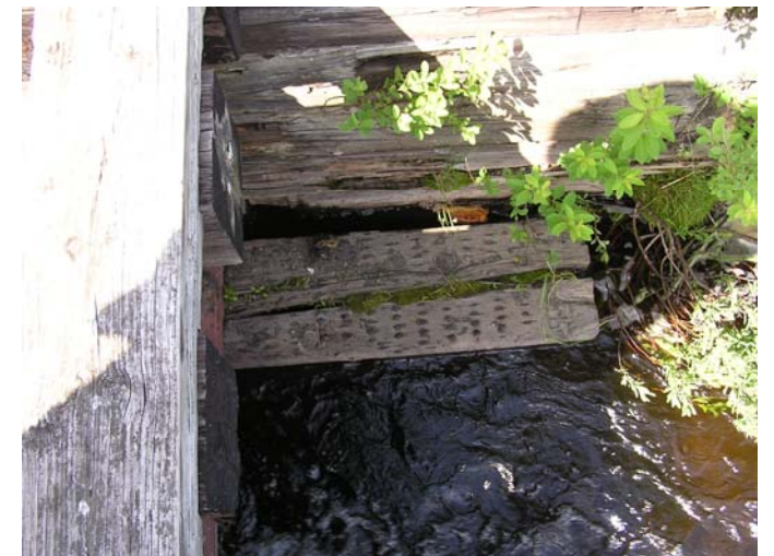
Figure 6-24 Bridge Over Round Pond Stream, top of timber abutment seat with split.
