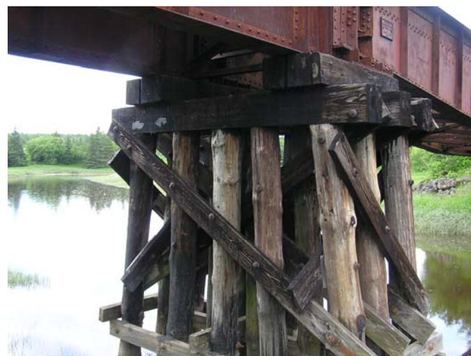
Figure 6-35 Bridge Over Little River, intermediate timber pier support.
