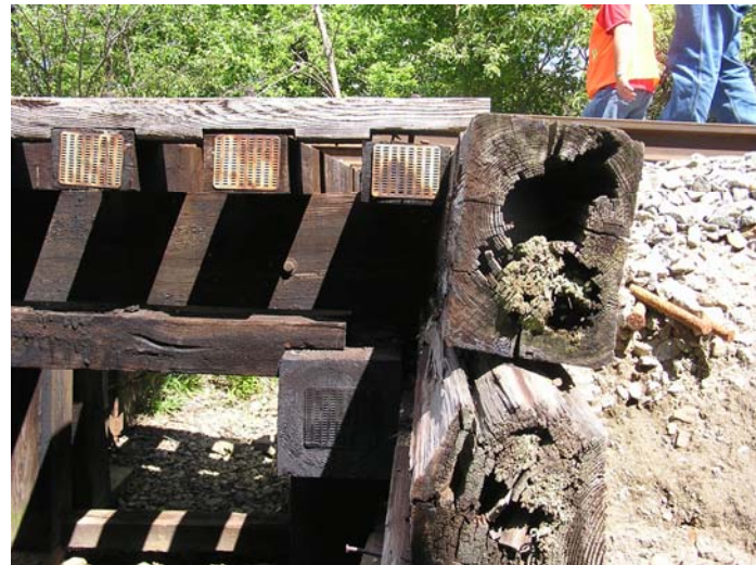
Figure 6-06 Cattle Pass. Note deterioration to timber backwall.
