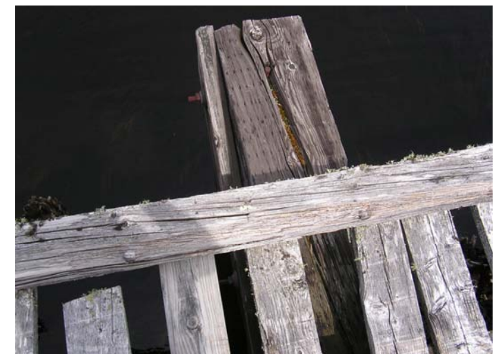
Figure 6-32 Bridge Over Pennamaquan River, typical condition of pile cap with deterioration.
