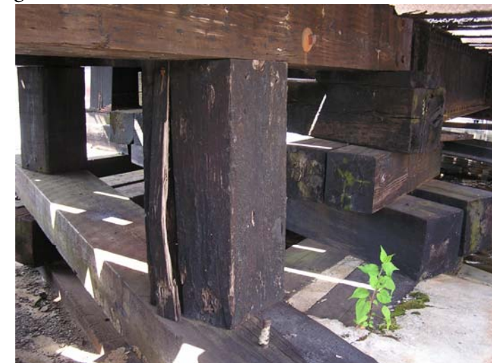
Figure 6-16 Salmon Falls International Bridge. Note crushing of timber post support, and decay in blocking.
