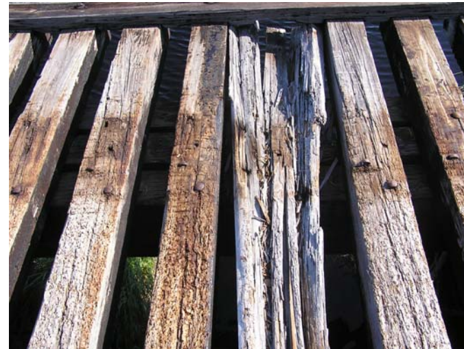
Figure 6-26 Bridge Over Ohio Brook, timber ties with severe deterioration.
