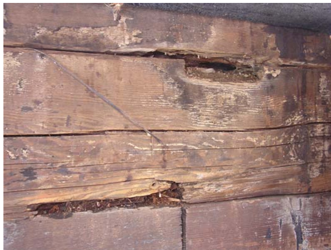
Figure 6-07 Cattle Pass. Note deterioration to timber backwall.
