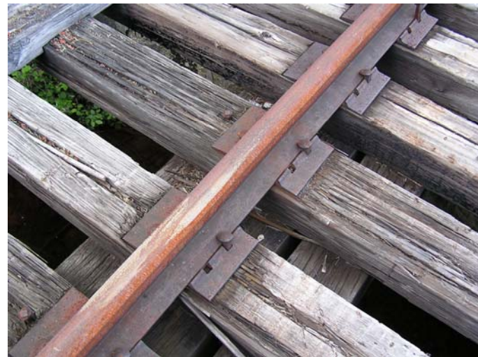
Figure 6-19 Bridge Over Moosehorn Brook. Note poor condition of the timber ties.
