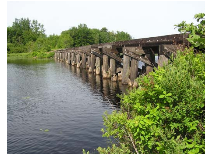
Figure 6-29 Bridge Over Pennamaquan River, looking west.
