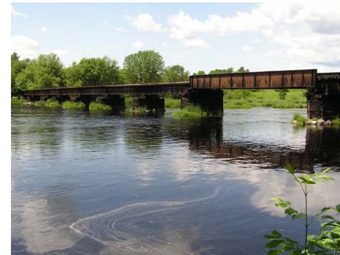
Figure 6-09 Baring International Bridge, looking south.
