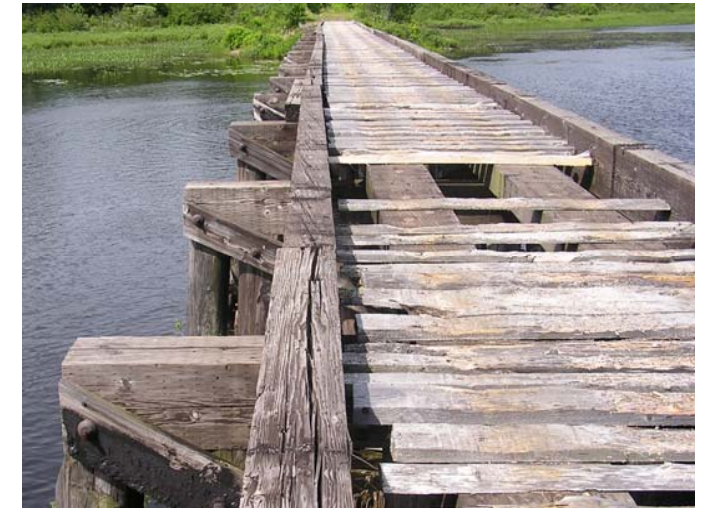
Figure 6-30 Bridge Over Pennamaquan River, top of deck. Note interior girders turned on their sides.
