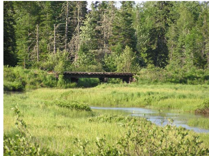
Figure 6-25 Bridge Over Ohio Brook, looking north.
