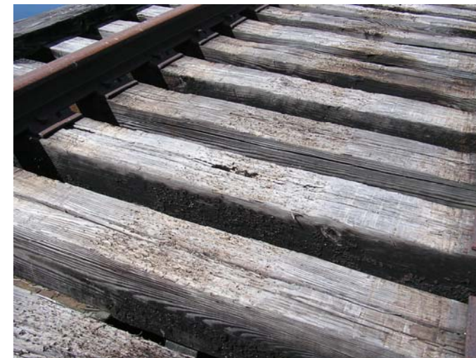
Figure 6-23 Bridge Over Round Pond Stream, timber ties.
