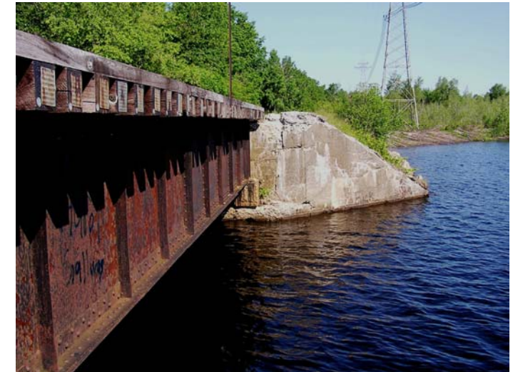
Figure 6-02 Sprague Falls International Bridge. Note severe deterioration to the abutment seat and wingwalls.
