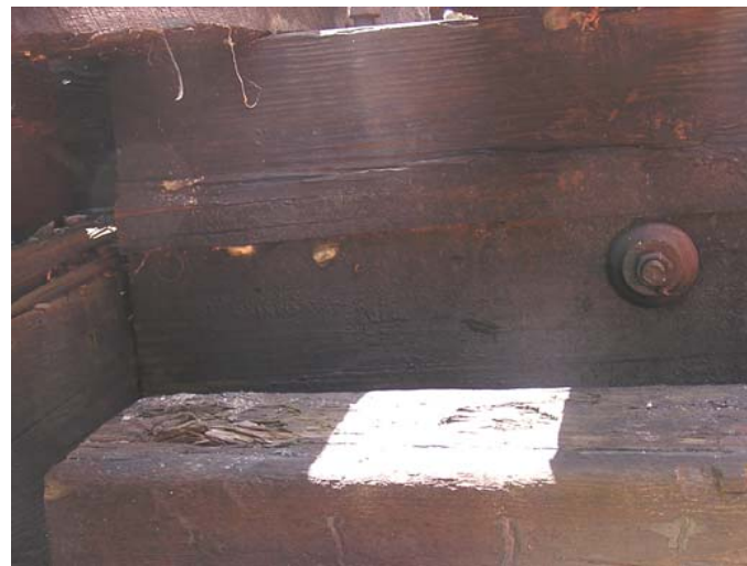
Figure 6-08 Cattle Pass. Note crushing/delamination of timber girder.
