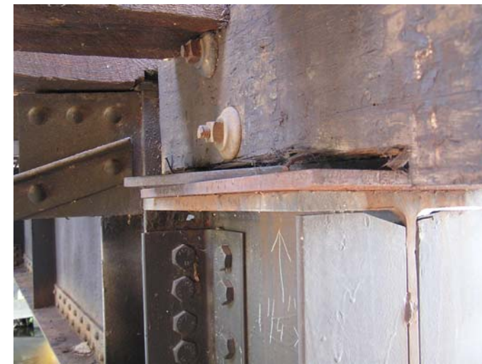
Figure 6-15 Salmon Falls International Bridge. Note rotated shims and new steel added to girder.
