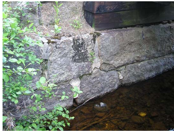
Figure 6-20 Bridge Over Moosehorn Brook, granite block abutments with pointing.
