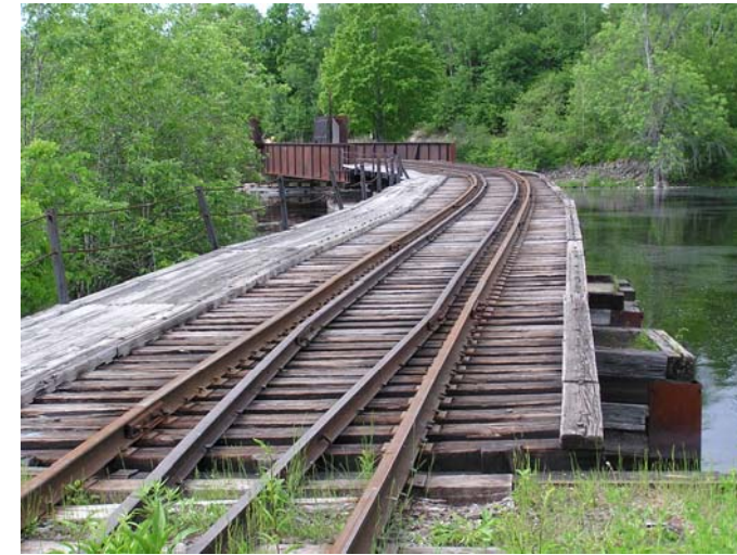
Figure 6-13 Salmon Falls International Bridge, looking south.
