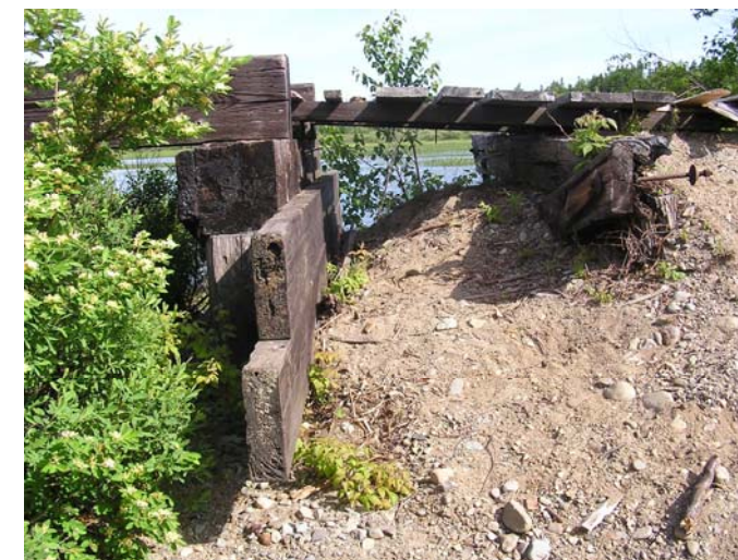
Figure 6-31 Bridge Over Pennamaquan River, depleted ballast and fill at backwall.
