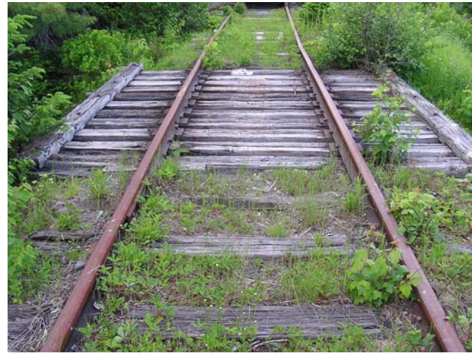
Figure 6-17 Bridge Over Moosehorn Brook, looking north.
