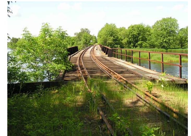
Figure 6-10 Baring International Bridge. Track view from U.S. approach.
