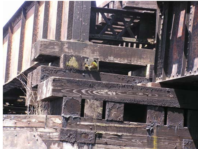
Figure 6-12 Baring International Bridge. Note crushing of timber post support, and deterioration in blocking.
