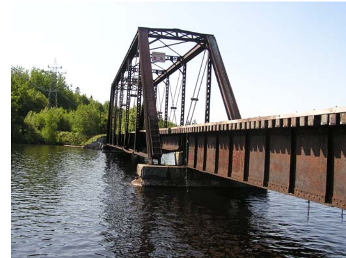
Figure 6-01 Sprague Falls International Bridge.
